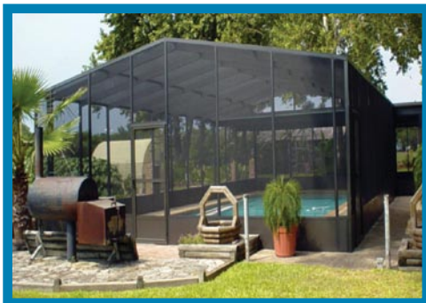
Right: Pool Cages can be free-standing as shown here on this Gable Roof pool cage. 2’ insulated kick plate is required for strength and provides a barrier for lawn debris.
