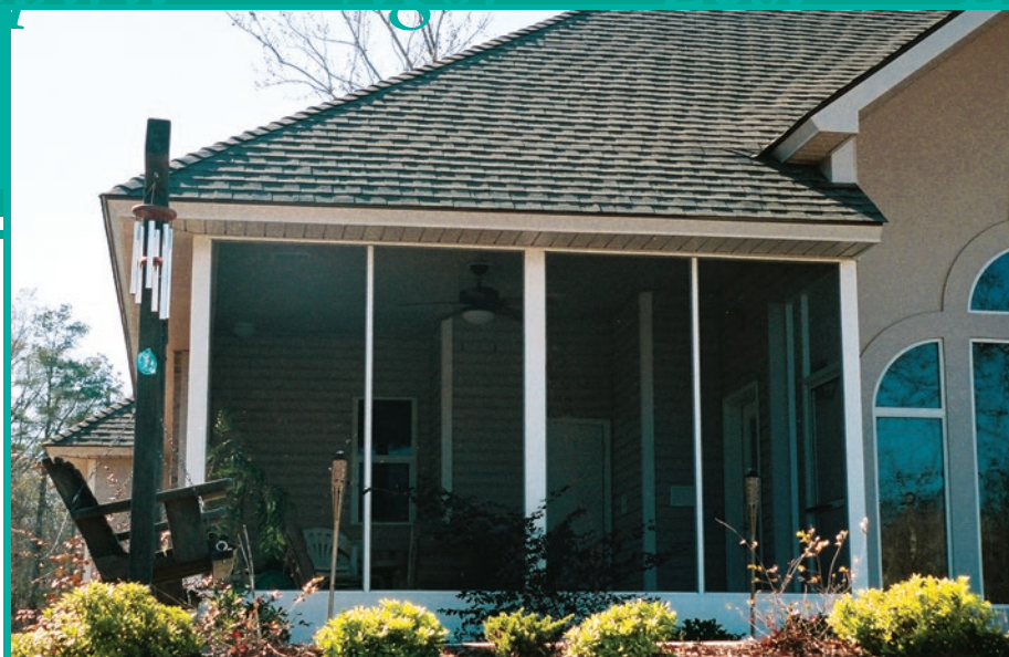
Above: This screen room is built around the existing structural aluminum post which supports the conventional roof of this house.
